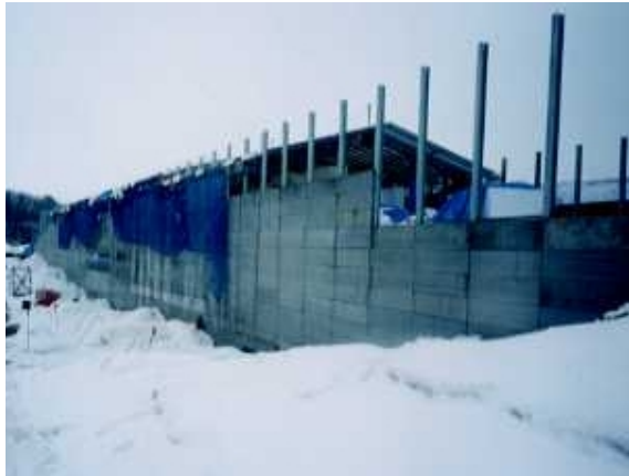
Photo-4. H-steel piles and facing
