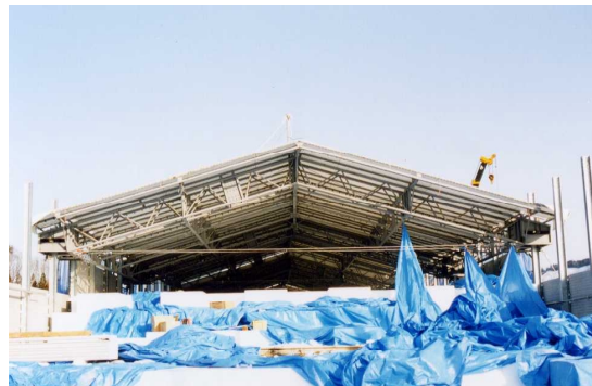
Photo-2. All-weather roofing system.
