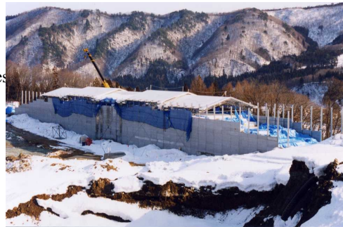
Photo -1. Overview of the site.
