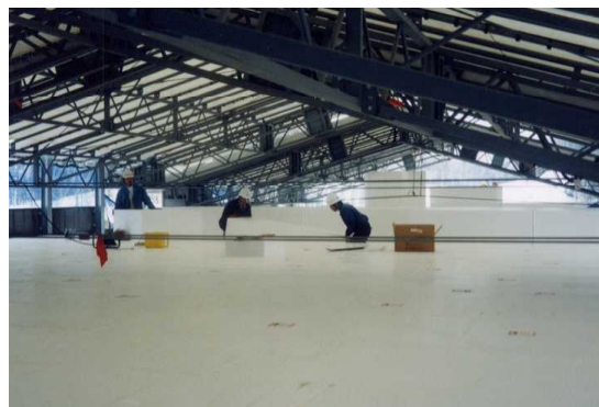
Photo-3. Installing the EPS blocks.
