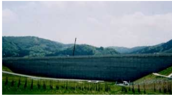
Photo-7. Completion of entire construction.
