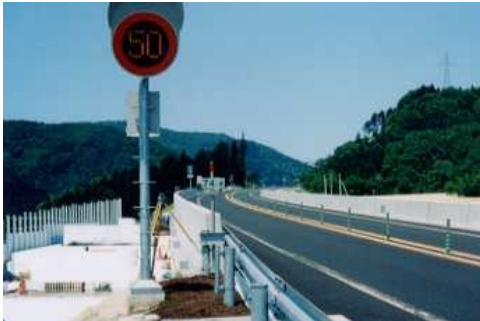
Photo-6. Completion of the 1st-period construction.
